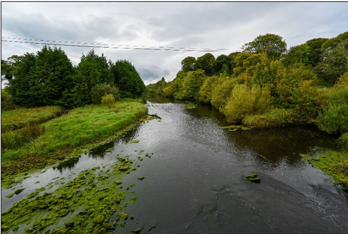
Plate 35 The 5 th order Cloonagmore river at Palmerstown Bridge. The proposed grid connection route crosses here. An Otter was seen at this site.
